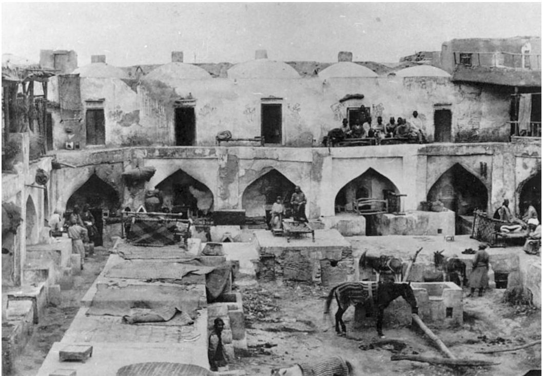
An Indian caravanserai in Bukhara, 1890s 16
