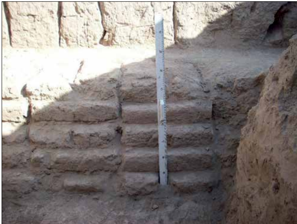
Fig. 65. Kultepa. Type of sufa laying in room 2.
