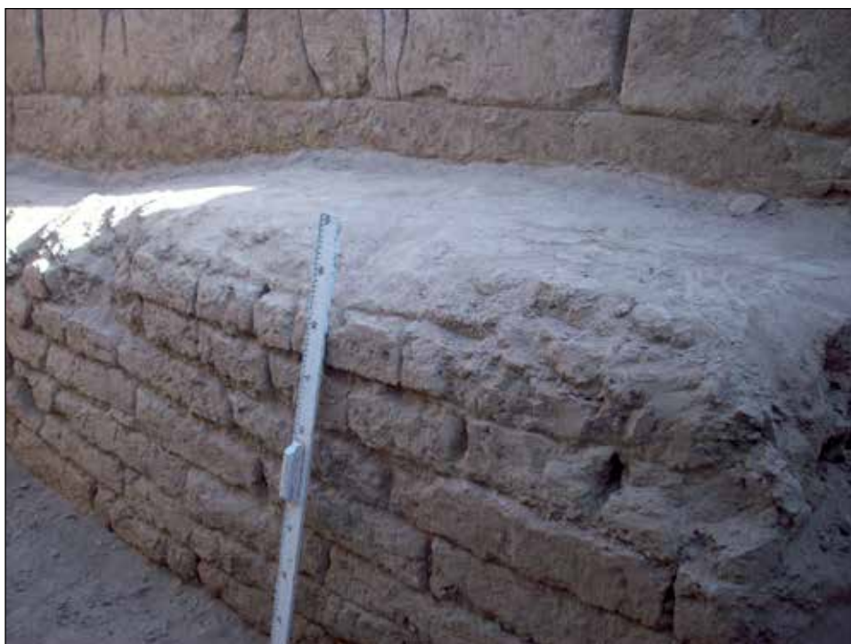
Fig. 62. Kultepa. Type of sufa laying in room 1.
